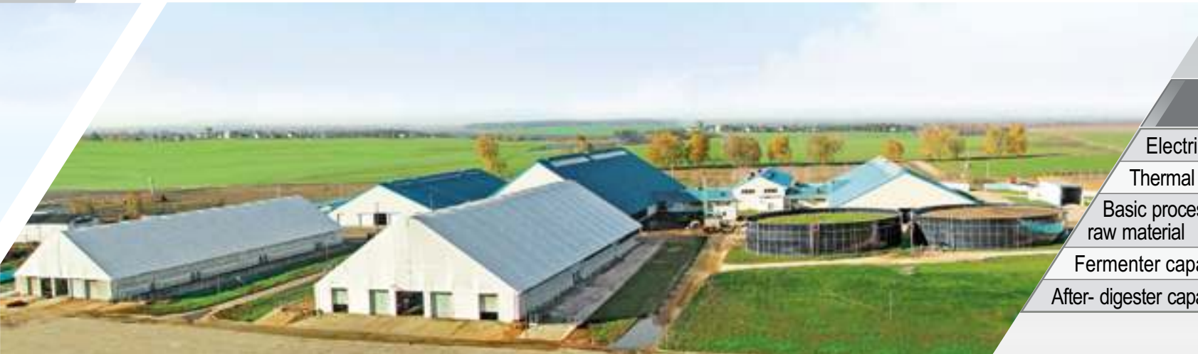
Biogas energy complex in Experimental Base "Zazerje" of the Scientific-Practical Center of the National of Academy of Sciences of Belarus for Agricultural Mechanization
